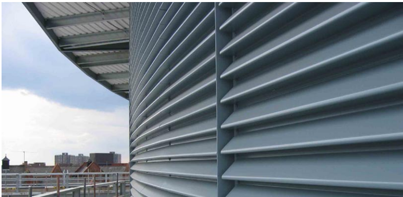
Typical APL non-combustible louvre profile assembly
